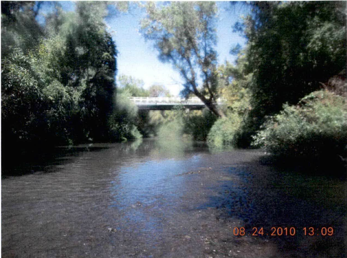
Figure C Looking upstream at the Highway 175 Bridge above the Hopland survey site.
